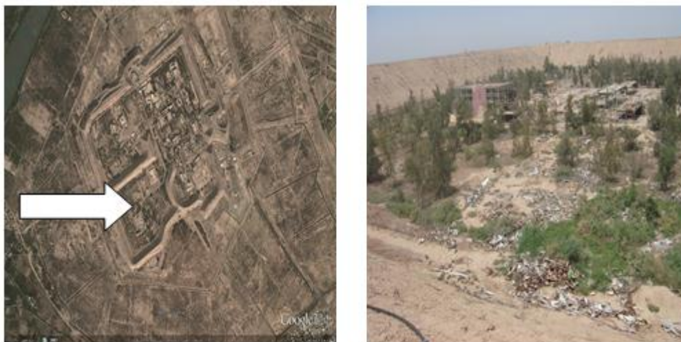
Fig. 1. Location of (FFF) inside Al-Tuwaitha site. Fig. 2. Shows the current condition of FFF
